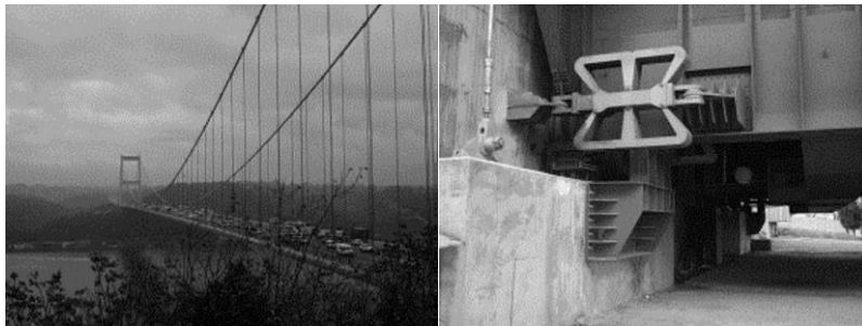
Figure 2-3. Second Bosphorus Bridge and facilities installed. Source: JICA
