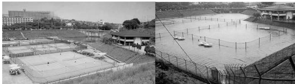
Figure 2-5. Alternative use of retarding pond in urban area. During normal (left) and flooding (right), Source: MLIT
