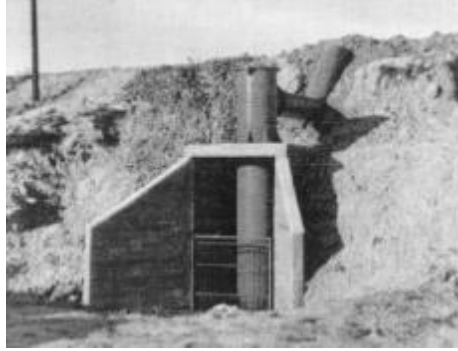
Figure 4.4. Flood control facility (water pump station) constructed just after the 1997-97 ENSO floods. Source: Salvatierra (2016)
