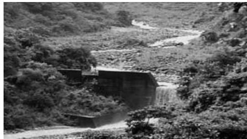
Figure 2-9. Sabo dam in Nepal. Source: JICA
