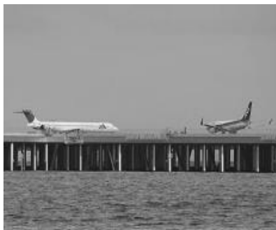
Figure 2-7. Tokyo Haneda Airport in consideration of flood risk mitigation. Source: Ishiwatari M.
