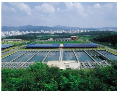
FIGURE 30: Sunnam Water Treatment Plant (786 m 3 /d) (K-water, 2015)
