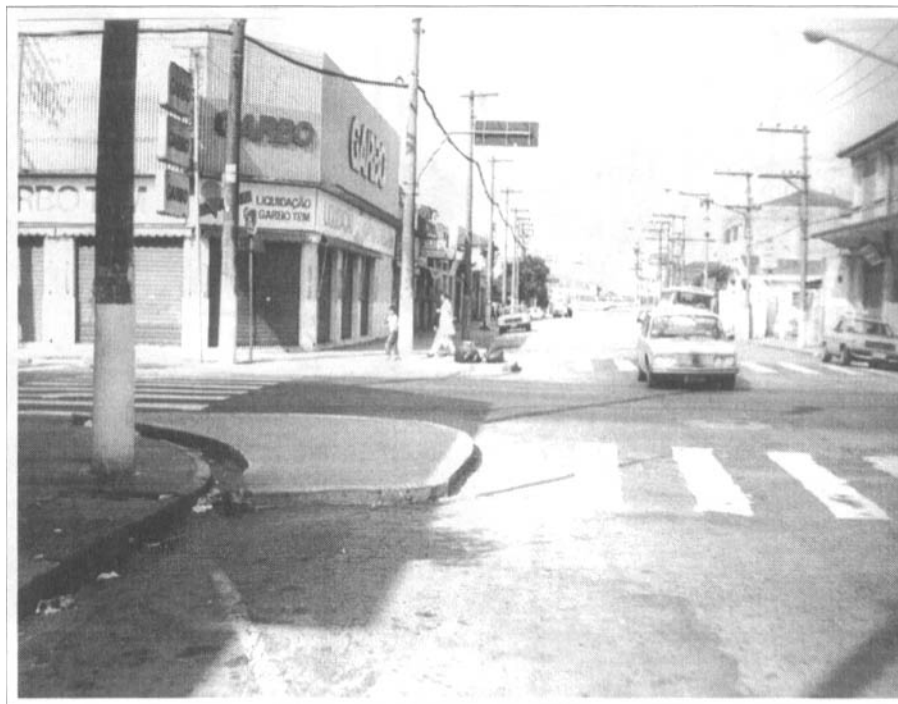
FIGURE 10.7 ENLARGEMENT OF SIDEWALK AT A CORNER SILVA BUENO STREET x COMANDANTE TAYLOR STREET– SÃO PAULO
