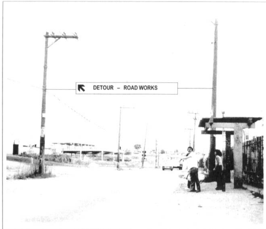
FIGURE 10.55 EXAMPLE OF THE USE OF BANNERS FOR TEMPORARY SIGNING
