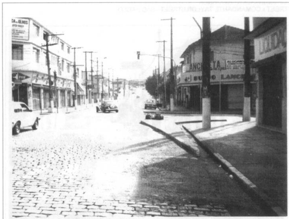
FIGURE 10.9 EXAMPLE OF GRADUAL NARROWING OF CARRIAGEWAY SILVA BUENO STREET x COMANDANTE TAYLOR STREET – SÃO PAULO
