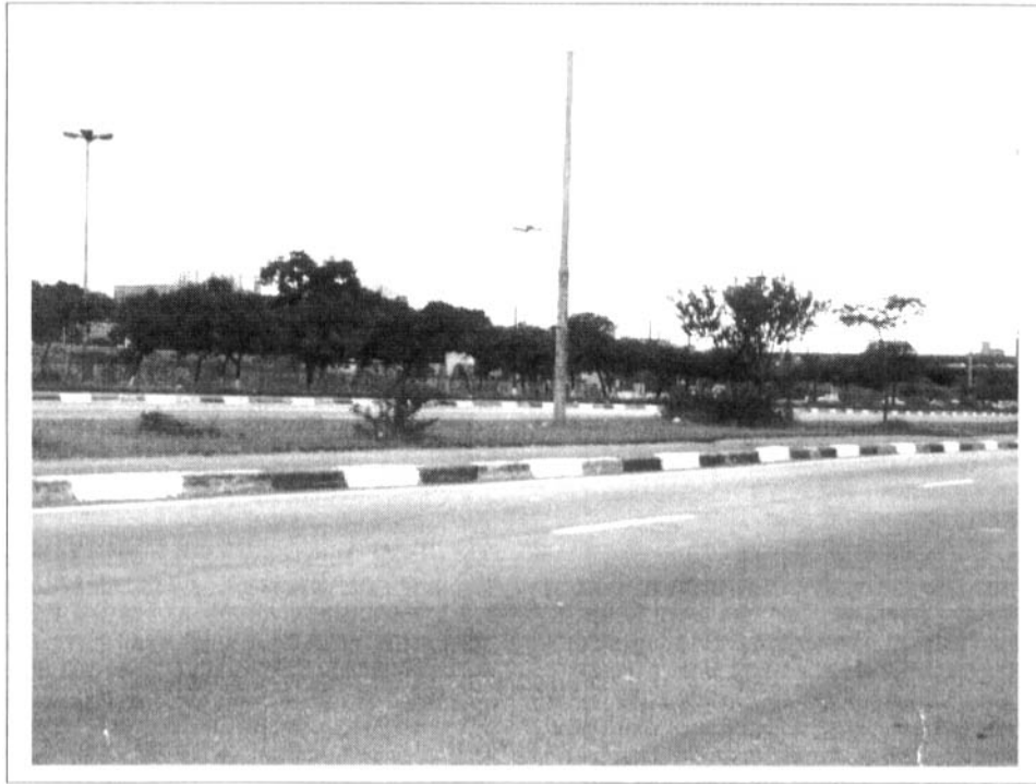
FIGURE 10.12 MEDIAN STRIP, SEPARATING VEHICLE FLOWS SALIM MALUF AVENUE – SÃO PAULO
