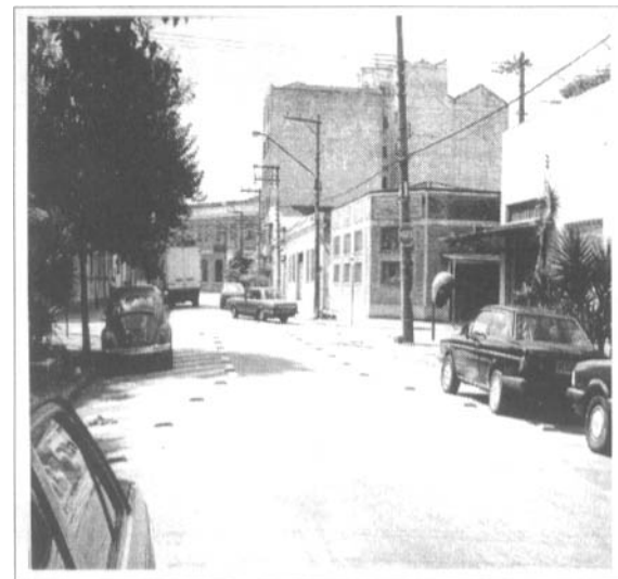
FIGURE 10.32 USE OF STUDS FOR ROAD NARROWING
