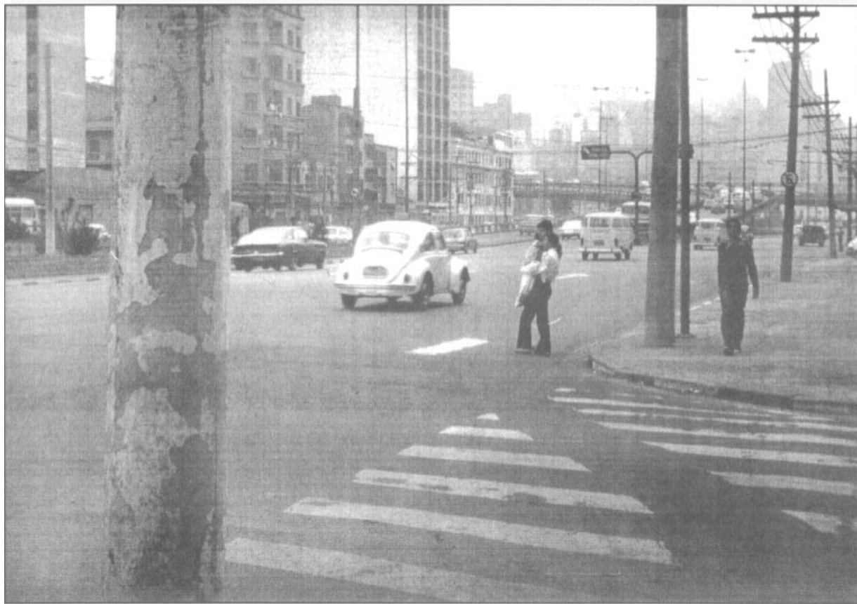
FIGURE 9.24 PEDESTRIANS CROSSING AT EF, MISLED BY REMAINS OF ROAD MARKING
