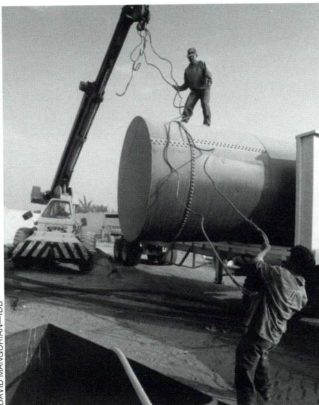
Building a fishmeal plant in Peru.
