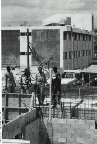
Hospital under construction.
