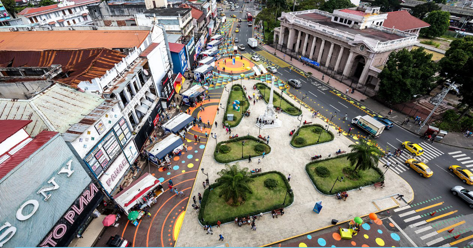
With the objective of transforming one of Panama City's most congested intersections into a less pedestrian-hostile place, the IDB supported the initiative "Panama Walks: Sharing Downtown" (PN-L1146).
