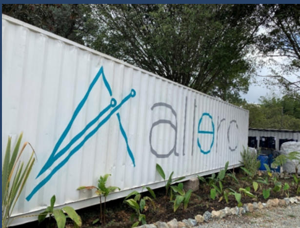
Figure 4-2: Modular ULIB recycling facility in Colombia
