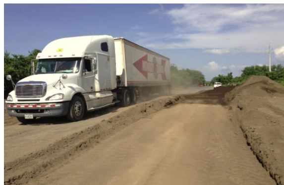
Figure 17: Landslides show road vulnerability to extreme weather events in Nicaragua
