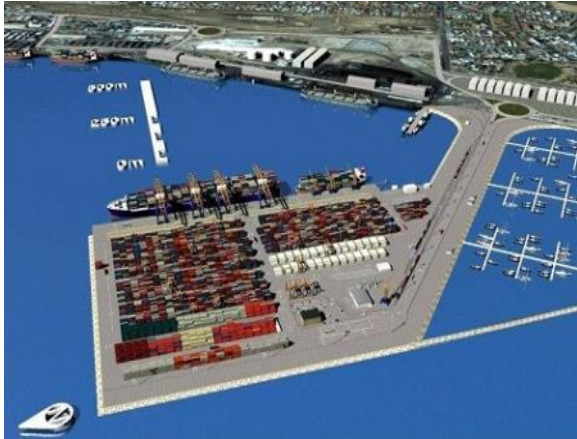
Figure 7: The Walvis Bay container terminal project, Namibia
