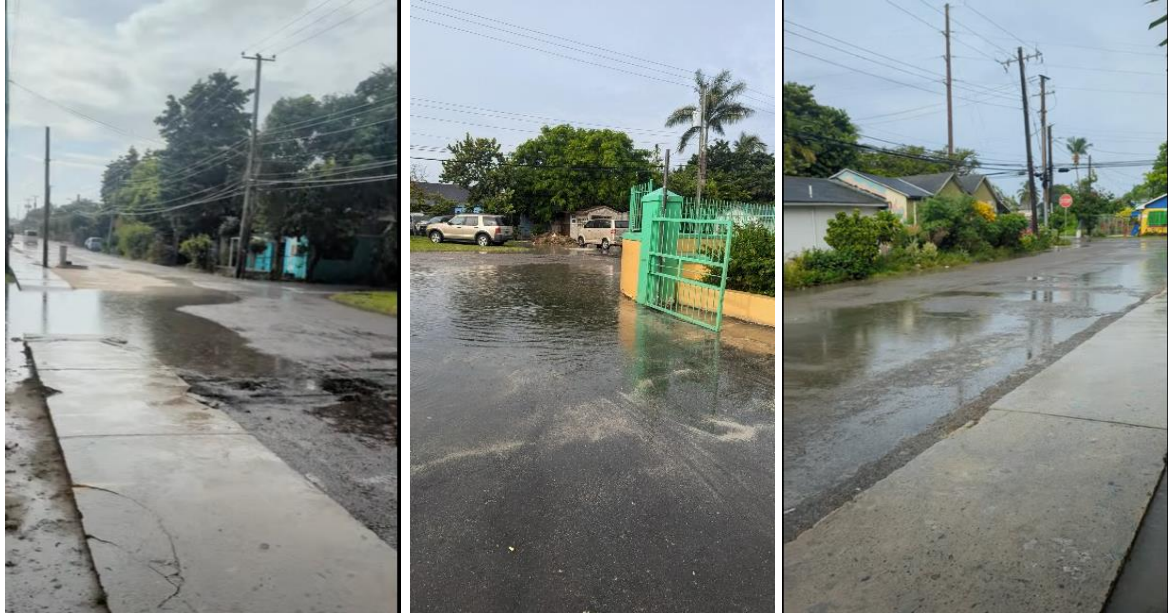
Figure 7. Flooding at the entrance of the Uriah McPhee Primary School
