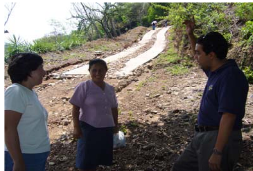
Pilot project to restore the road in the community
