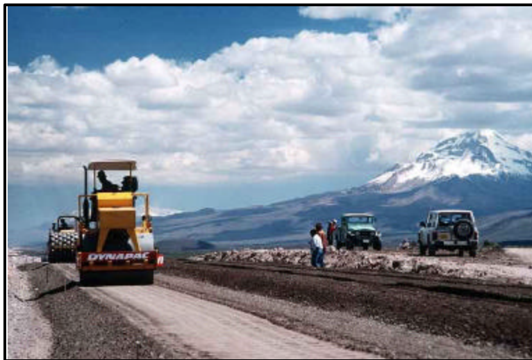
Road Construction in Bolivia
