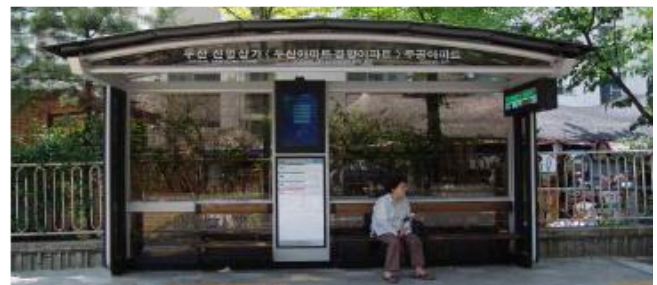
Figure 7 Open type platform
