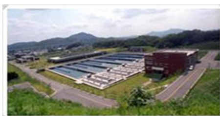
Integrated water treatment plant
