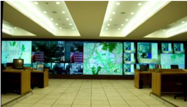
Figure 18 Anyang smart city center
