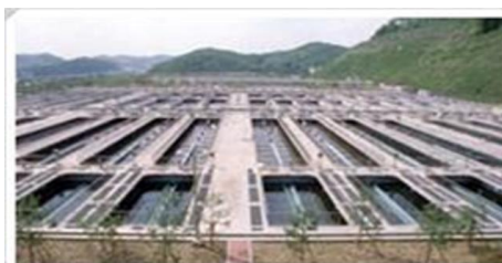
Sewage treatment plant
