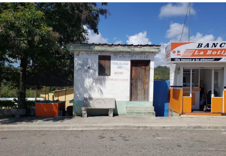
Illustration 15: Customer service and fee payment office in Los Montones, San José de las Matas. Source: SIASAR.
