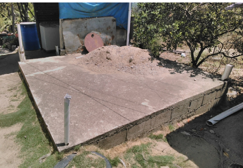
Illustration 11: Construction of a new installation over a pit. Source: CORAASAN household survey.
