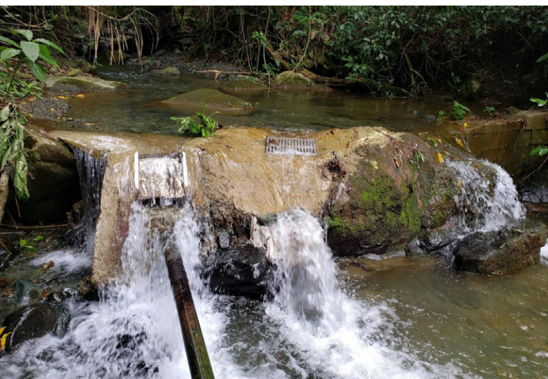
Illustration 13: Example of surface catchment in the Las Piedras gravity flow water supply systems in San José de las Matas. Source: SIASAR.
