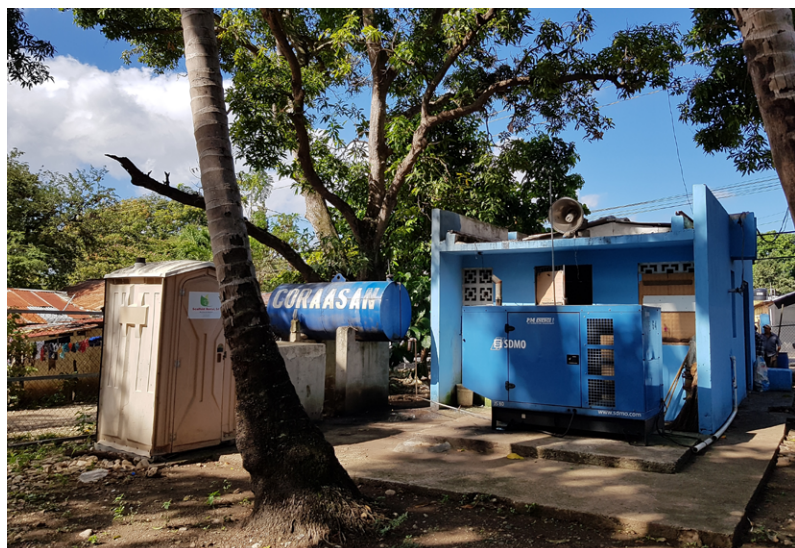
Illustration 14: Example of underground catchment by electric pumping managed by CORAASAN in Los Cocos, municipality of Santiago de los Caballeros. Source: Authors' preparation.
