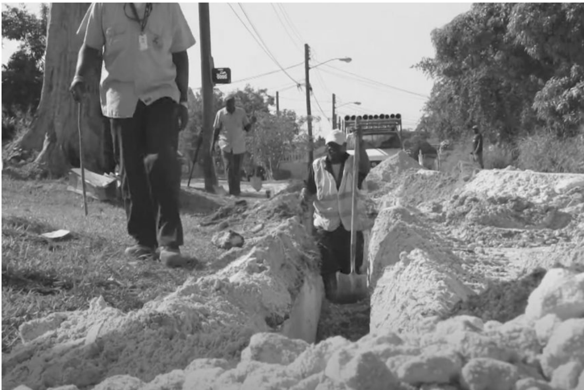
Workers excavating a trench for the installation of water pipes.
