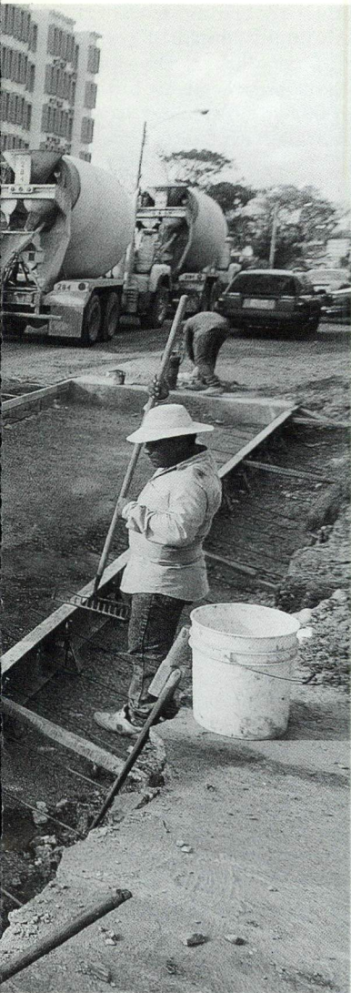
road rehabilitation project.
