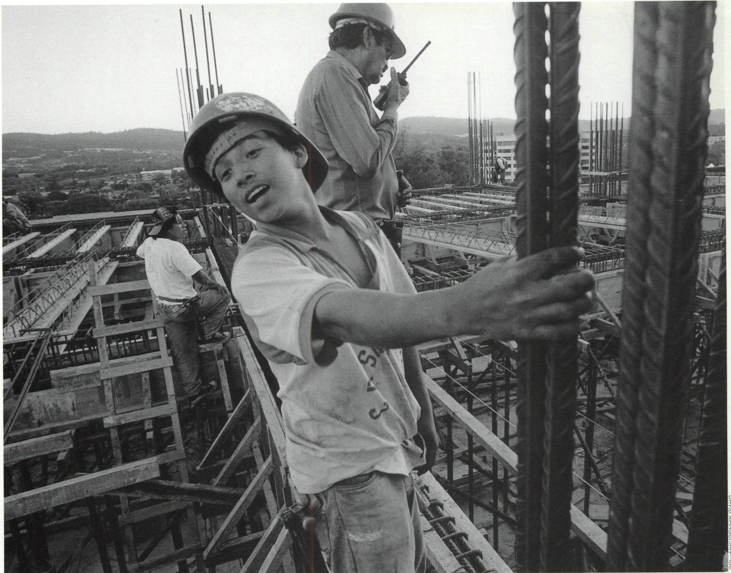
HIGH-LEVEL JOB: A young construction worker in San Salvador, El Salvador, gets a good grip on the reinforcing rods that will support the framework for a new hotel. The project was carried out with the help of an IDB-financed credit program.
