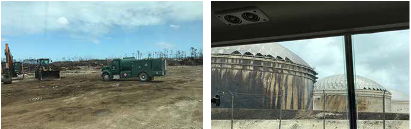
FIGURE 8. GRAND BAHAMA - OIL SPILL AT EQUINOR SOUTH RIDING OIL TERMINAL
