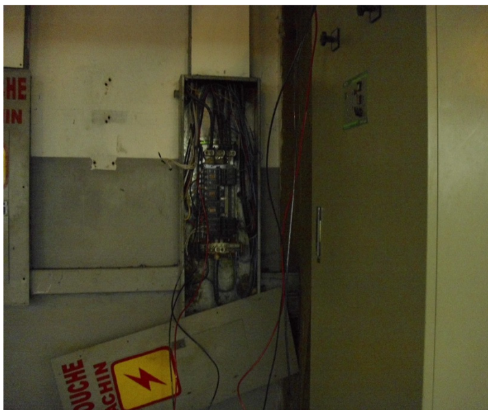
Figure 1. This electrical panel represents a possible ignition source as well as a potential source of shock or electrocution to workers.
