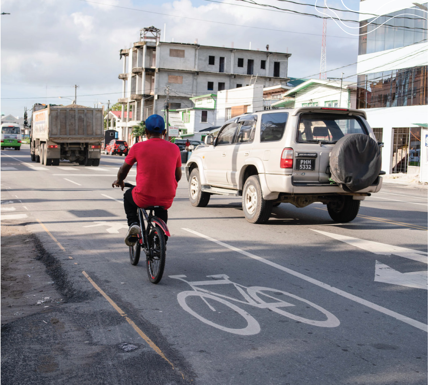
As part of upgrade to the Sherriff Street-Mandela roadway, sidewalks were installed as well as pedestrian crossings.
