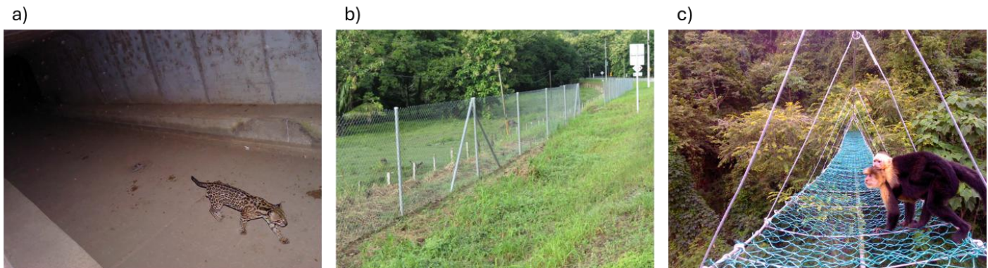
Fig. 2. Example of a) an underpass (square culverts with dry ledges for wildlife), b) fencing associated with the underpasses, and c) canopy bridges installed on Route 160.
