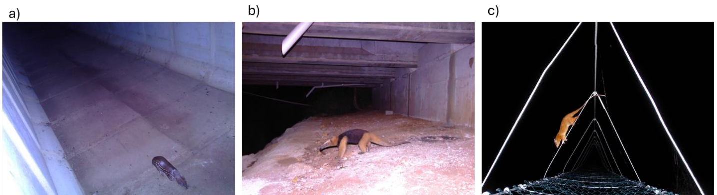
Fig. 3. Examples of a) box culvert, b) bridge adapted with ledges for wildlife, and c) canopy bridge installed on Route 1.
