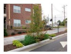
A tree box filter is a concrete box containing porous soil media and vegetation that functions like a small bioretention area but is completely lined, must have an underdrain, and has one or more trees. Runoff is directed from surrounding impervious surfaces to the tree box filter where it percolates through the soil media to the underlying ground. If the runoff exceeds the design capacity of the tree box filter, the underdrain directs the excess to a storm drain or another device.
