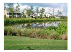
Wet ponds are constructed basins that have a permanent pool of water throughout the year (or at least throughout the wet season). Also called stormwater ponds, retention ponds, and wet extended detention ponds, they differ from constructed wetlands primarily in having a greater average depth. The primary removal mechanism is settling, as stormwater runoff resides in this pool. Limited pollutant uptake, particularly of nutrients, also occurs to some degree through biological activity in the pond.
