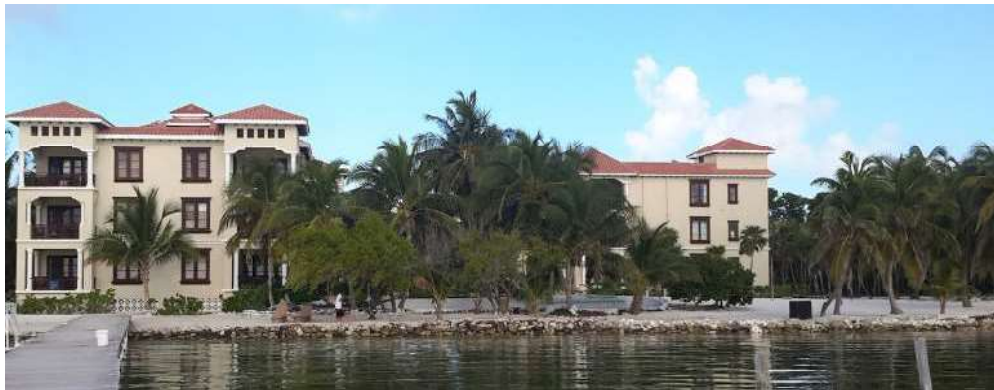
Figure 12. Rip-rap seawall on the northern end of Ambergris Caye North PHS.
