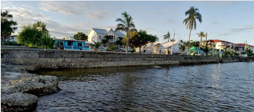
Figure 7. Seawall on the northern half of Corozal PHS.
