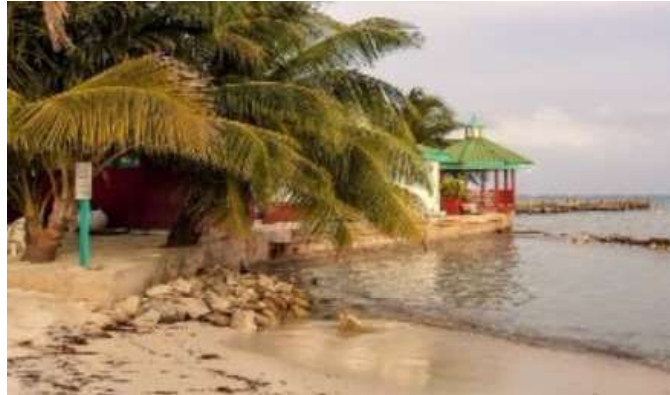
Figure 19. Vertical Seawall and Rip-Rap Protection in San Pedro (Belize).
