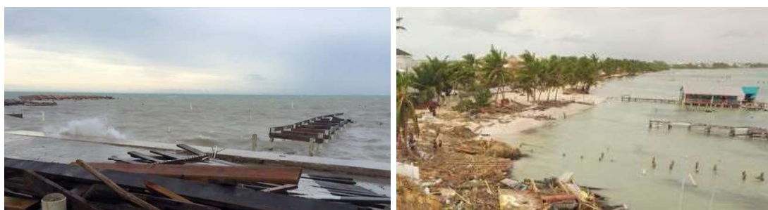
Figure 21. Seawall and beach in San Pedro right after Hurricane Earl (2016).
