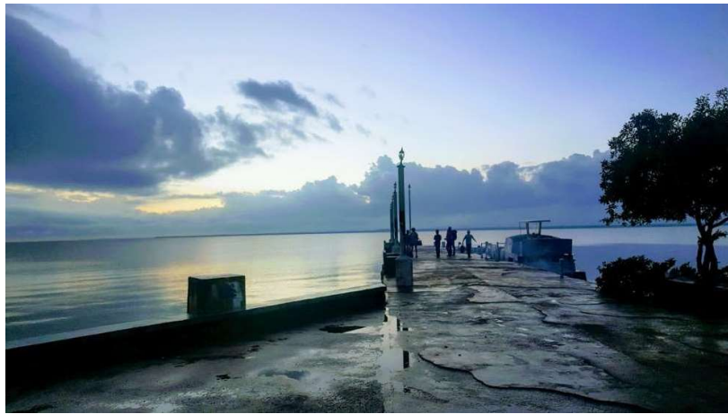
Figure 6. Mooring dock on the northern end of Corozal PHS.
