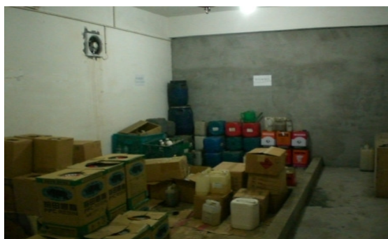
Figure 2. Two examples of secondary containment for chemical storage. On the left, the berm structure raised above the floor is part of the room construction. On the right, a stand-alone secondary containment device. It should be noted that the quantity and arrangement of containers in the photograph on the left may not represent safe conditions.
