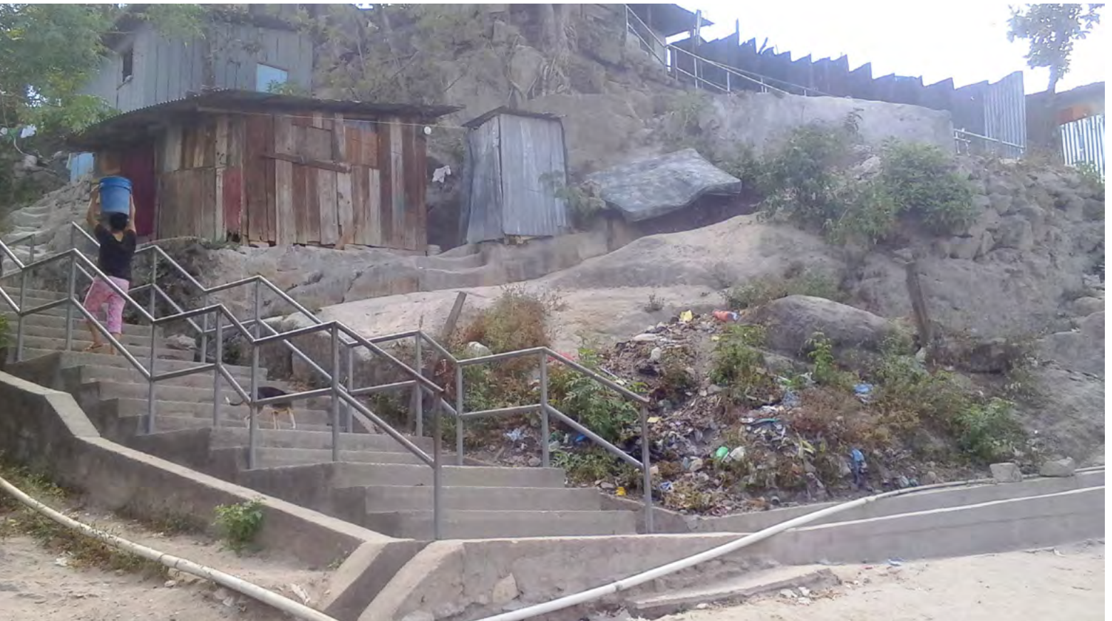
Photo 3: Woman carrying pail of water in newly built stairs, Los Pinos
