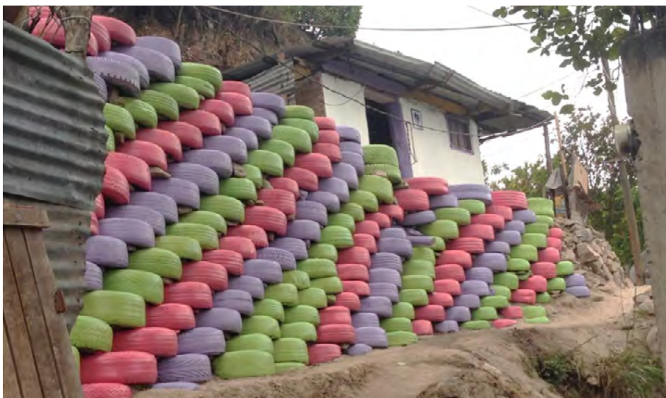
Photo 19: Building the new tire wall, Villa Nueva
