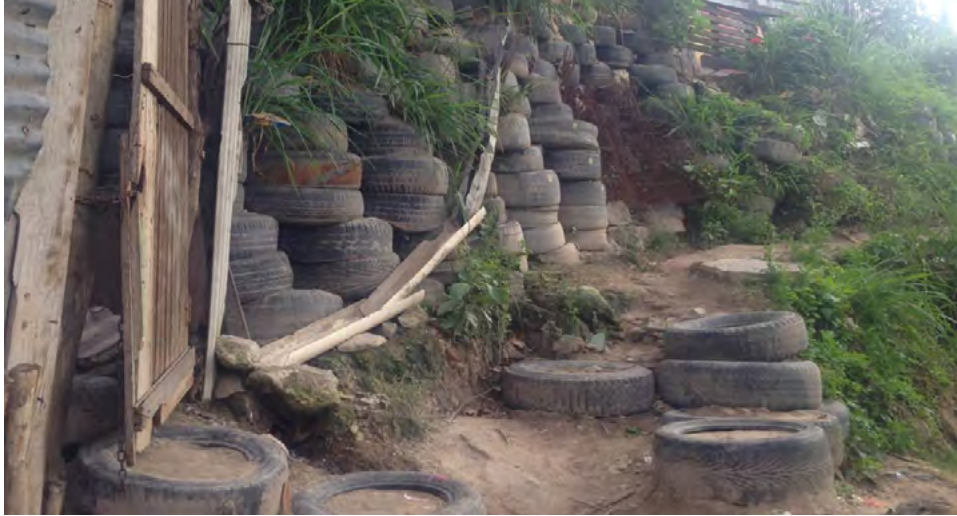
Photo 18: The existing tire wall, Villa Nueva
