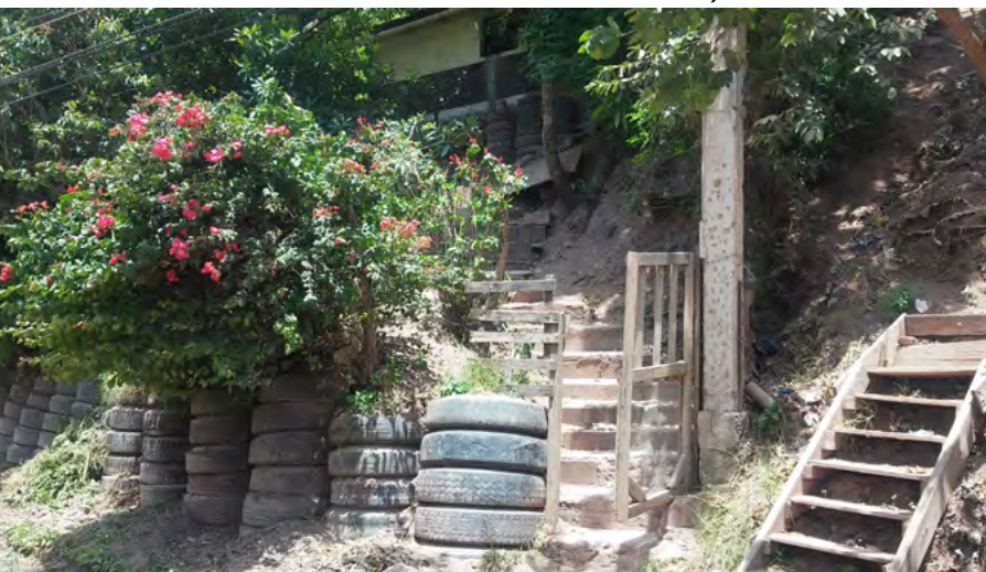
Photo 15: Retention wall with used tires, Los Pinos
