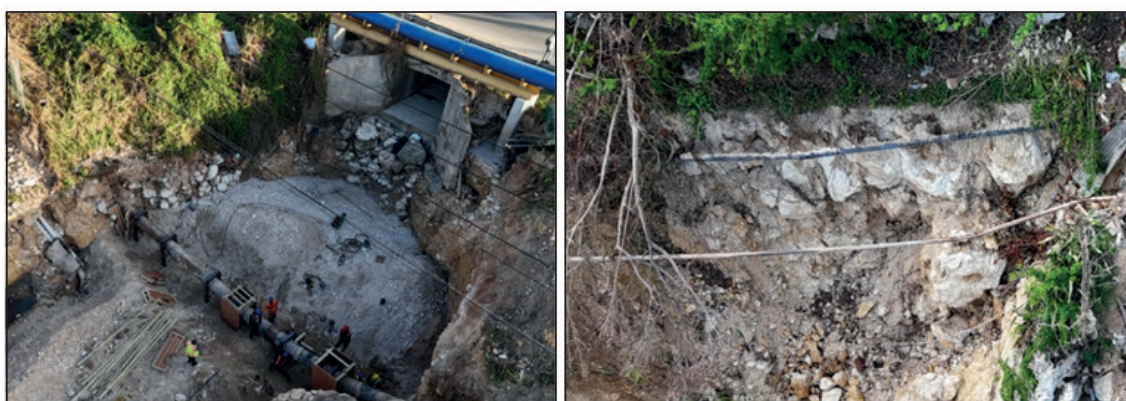
Pipeline repairs to transmission main through the Lilliput Gulley
