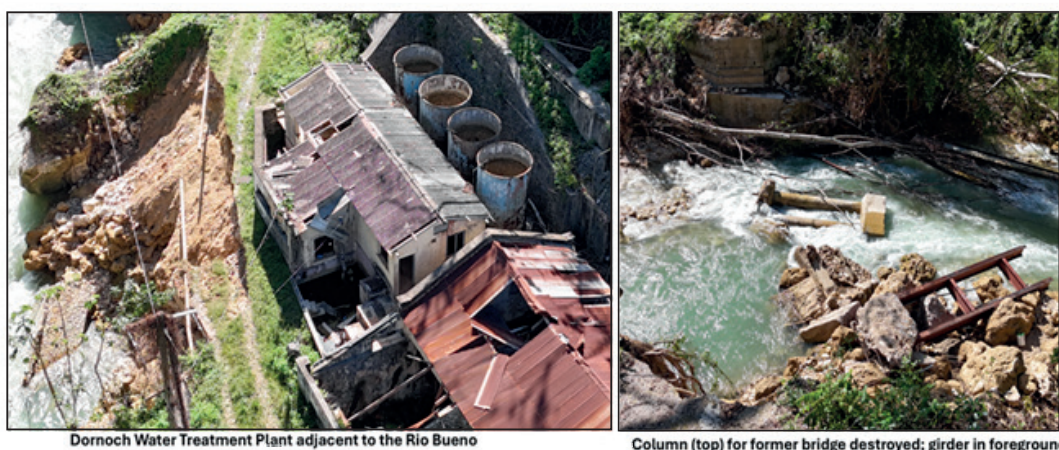
Dornoch Water Treatment Plant adjacent to the Rio Bueno
