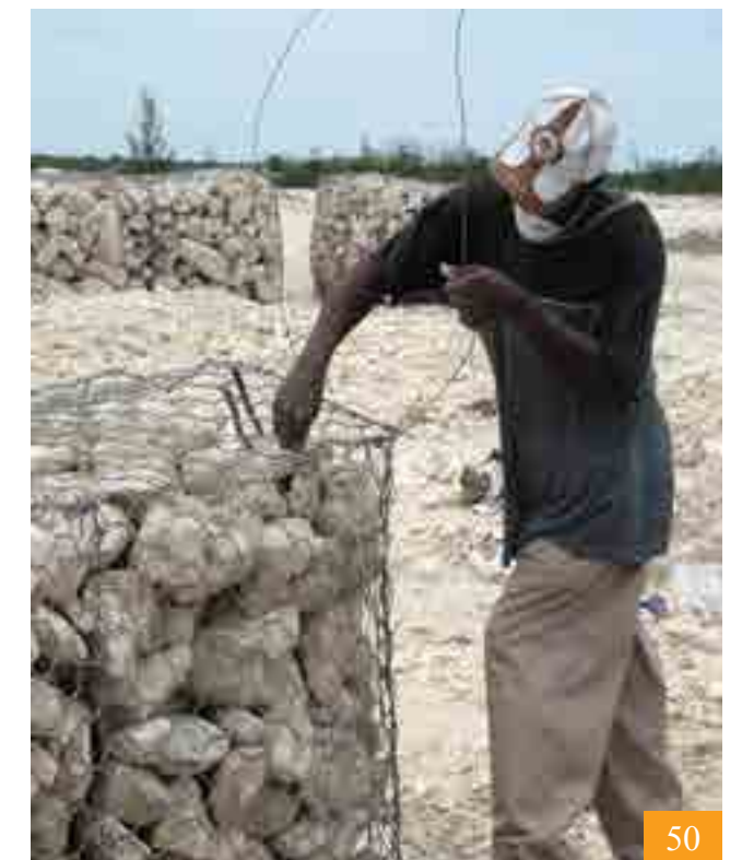
NASSAU, BAHAMS. CONSTRUCTION OF GABION BASKETS. JUNE, 2004
