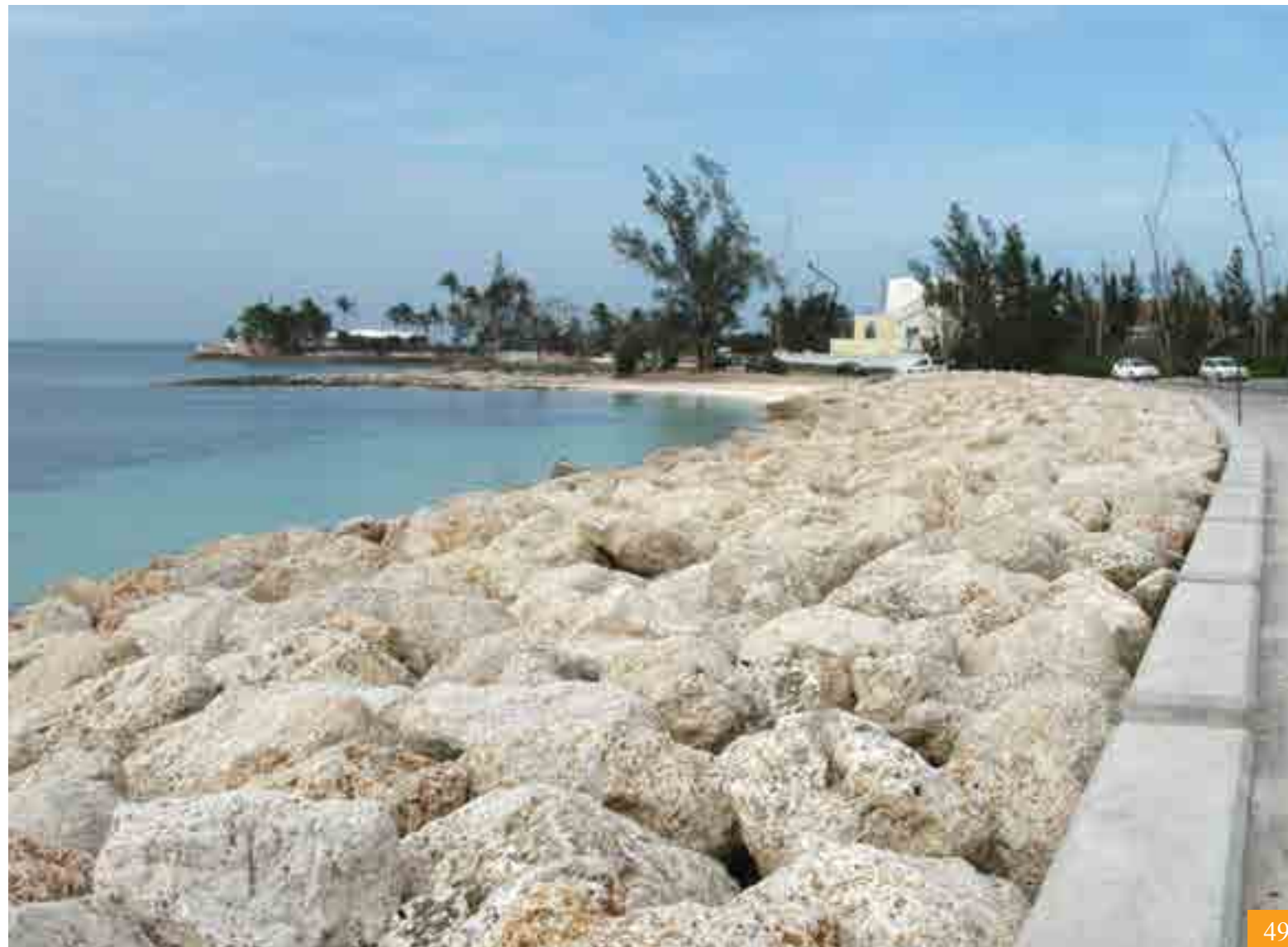
NASSAU, BAHAMAS. BREAKWATER. JUNE, 2004
