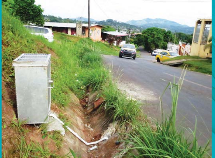
Monitoring point in La Alameda (AL) with negative pressures.
