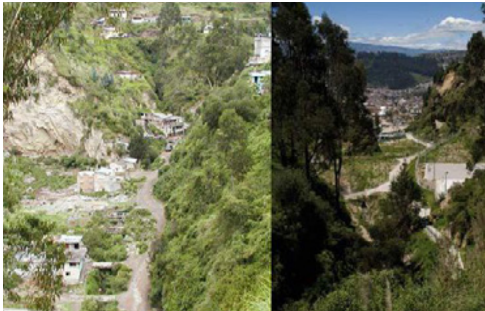
Figure 11: Jerusalén Ravine project / Left before works - Right after works
