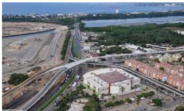
Manzanillo Port elevated roadway building program
