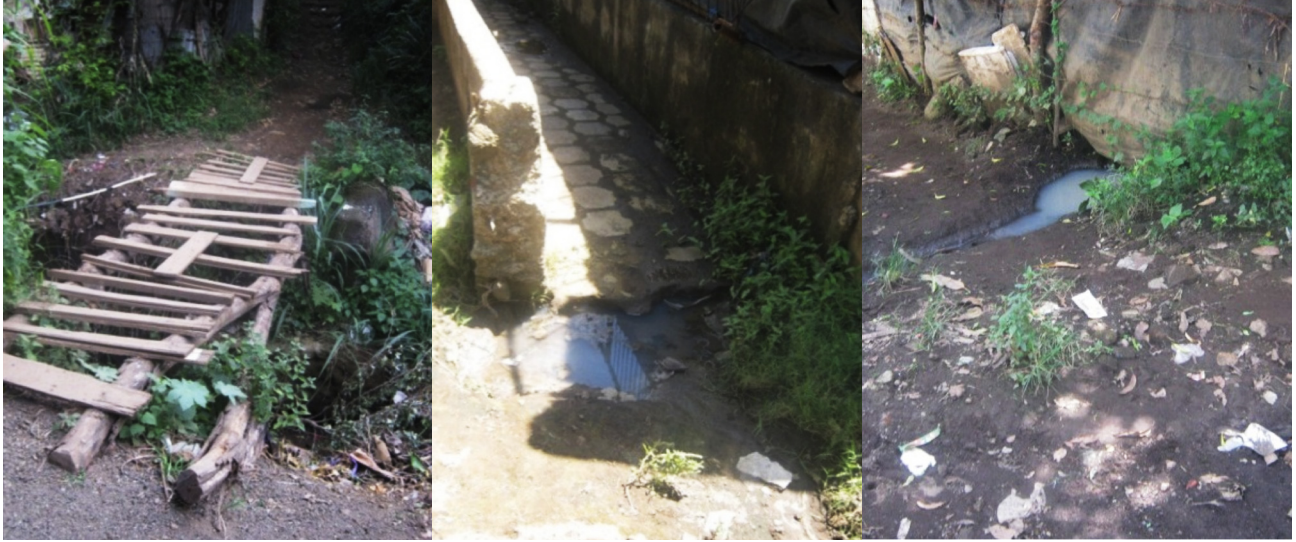
Figure 4-3: Neighborhood infrastructure in need of repair
