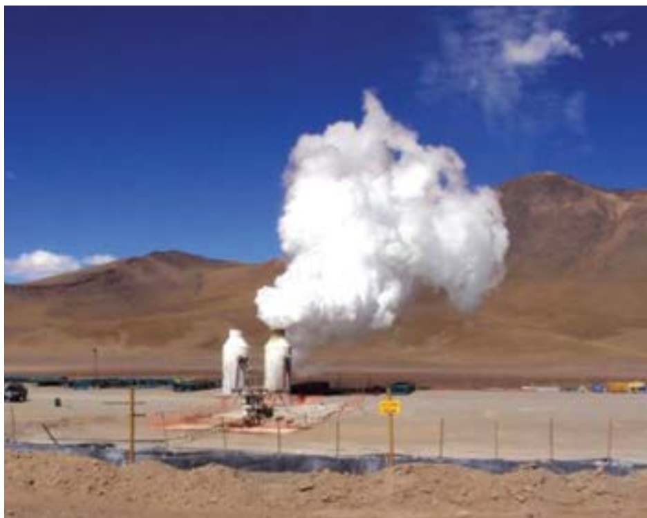
Testing of Cerro Pabellón geothermal wells.
