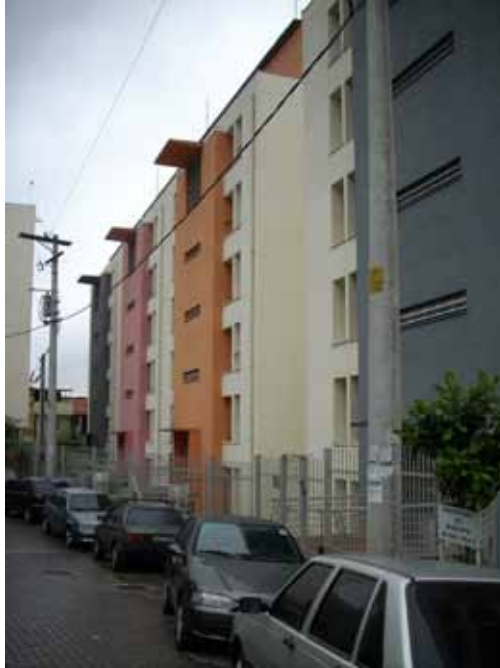
Cingapura/PROVER in São Paulo – 2nd phase
